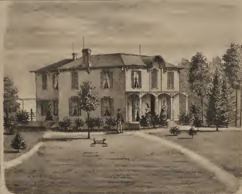
RESIDENCE OF K. N. LEACH, FOUNTAIN GREEN, ILL.
